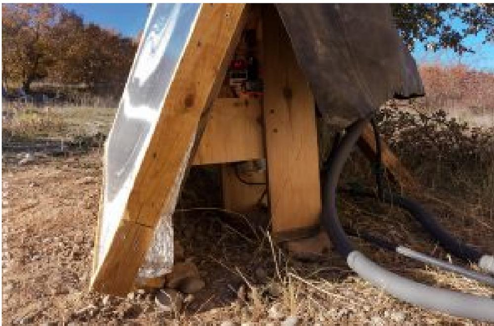
Pump, thermostat and thermometers are installed at the back of the solar panel. The tubes are insulated with foam rubber socks. The front of the panel is covered with a sheet of plexiglass. 28 November 2017.
