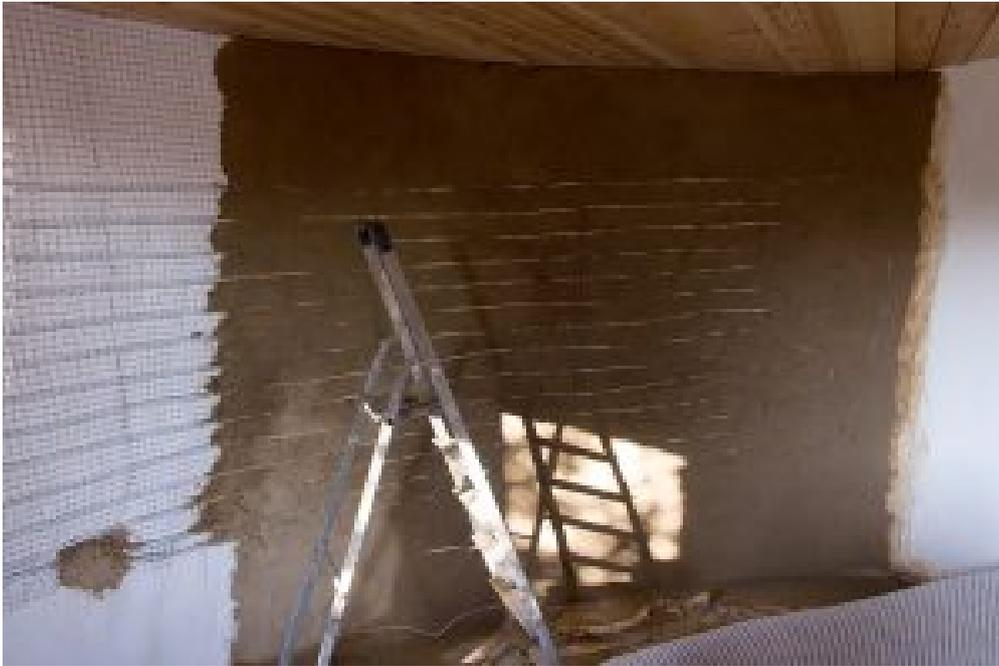
Applying the clay mix with a trowel. Before applying I sprayed abundant water and once applied it is important to let it dry completely before starting with the next layer. 4 October 2017.
