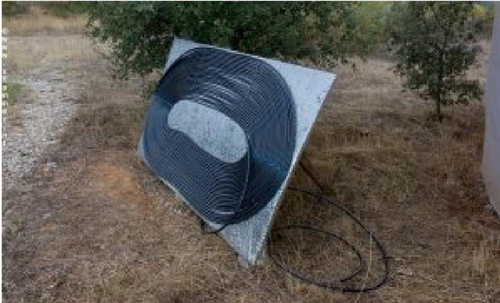
The DIY solar panel, just two meters separated from the interior tube system and exposed to the south. It measures about 2 x 1 meter and gives support for 100 meters of black irrigation tube. 18 September 2017
