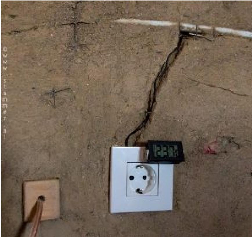
This digital thermometer, installed on an electricity socket, is connected with its sensor close to the heating tube. After whitewashing the wall it's the only element noticeable of the heating system inside. It keeps track of the temperature near the point of entrance where the water is hottest. On a typical sunny winter day it stabilizes around 28°C. 30 October 2017.
