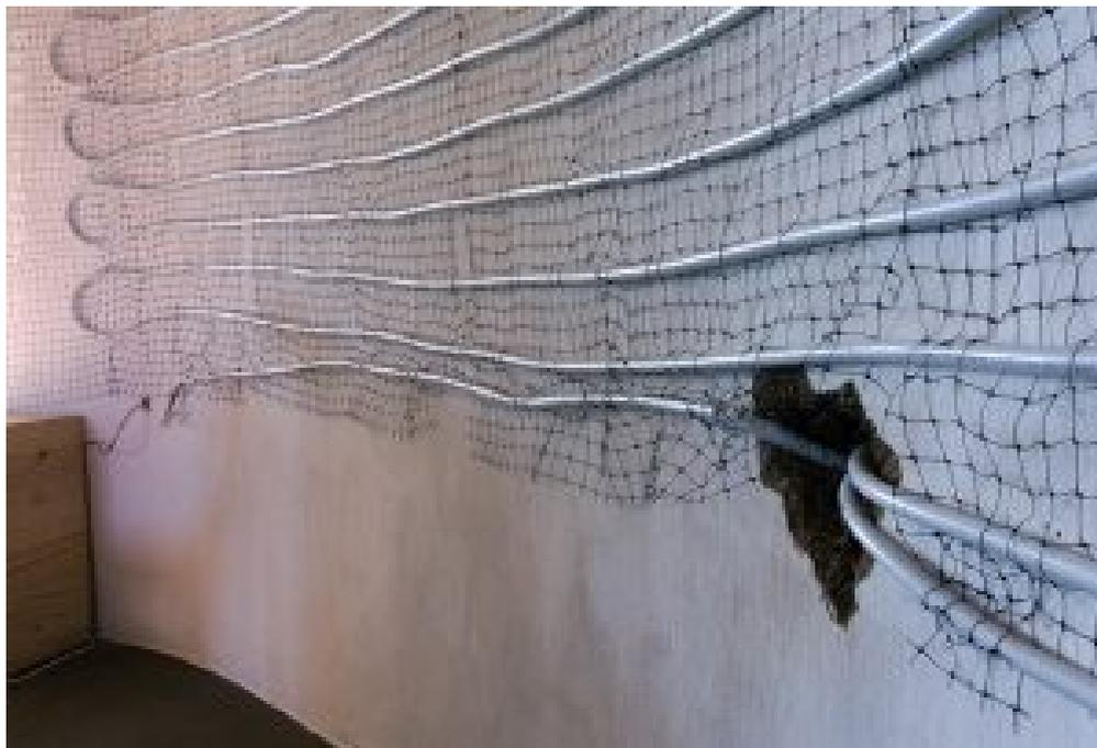
It took me almost two days to sew the 100 meter heating tube into the nylon net, but in combination with more than 1000 staples the installation is perfect. 27 September 2017.
