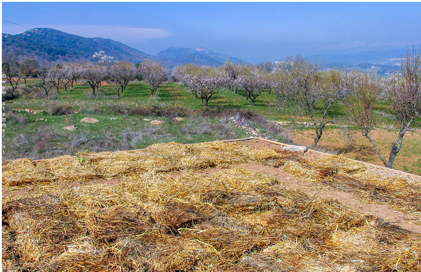
March 2009. The 'strawbooks' are spread out onto the soil and Sedum cuttings are planted between them.
