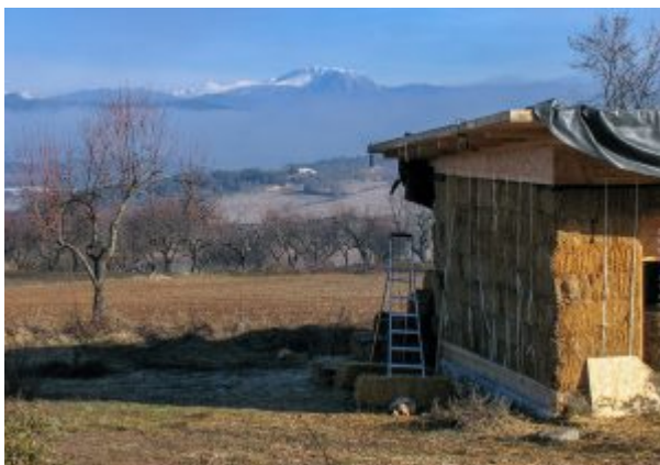
January 2009. The roof of the first straw bale module is ready and the first layer, the EPDM sheet, has been spread out.
