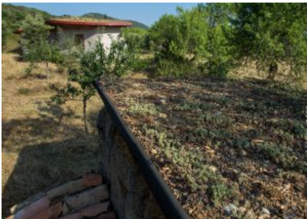
July 2018. The Sedum roof of the compost toilet building.
