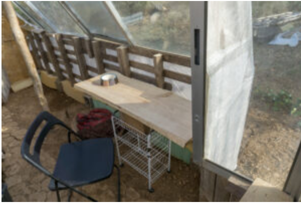
Foam and concrete blocks insulate the pallets from the soil. The metal mesh is also fixed with staples.
