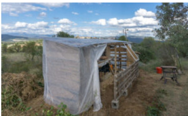
The geotextile cloth is fixed with staples.
