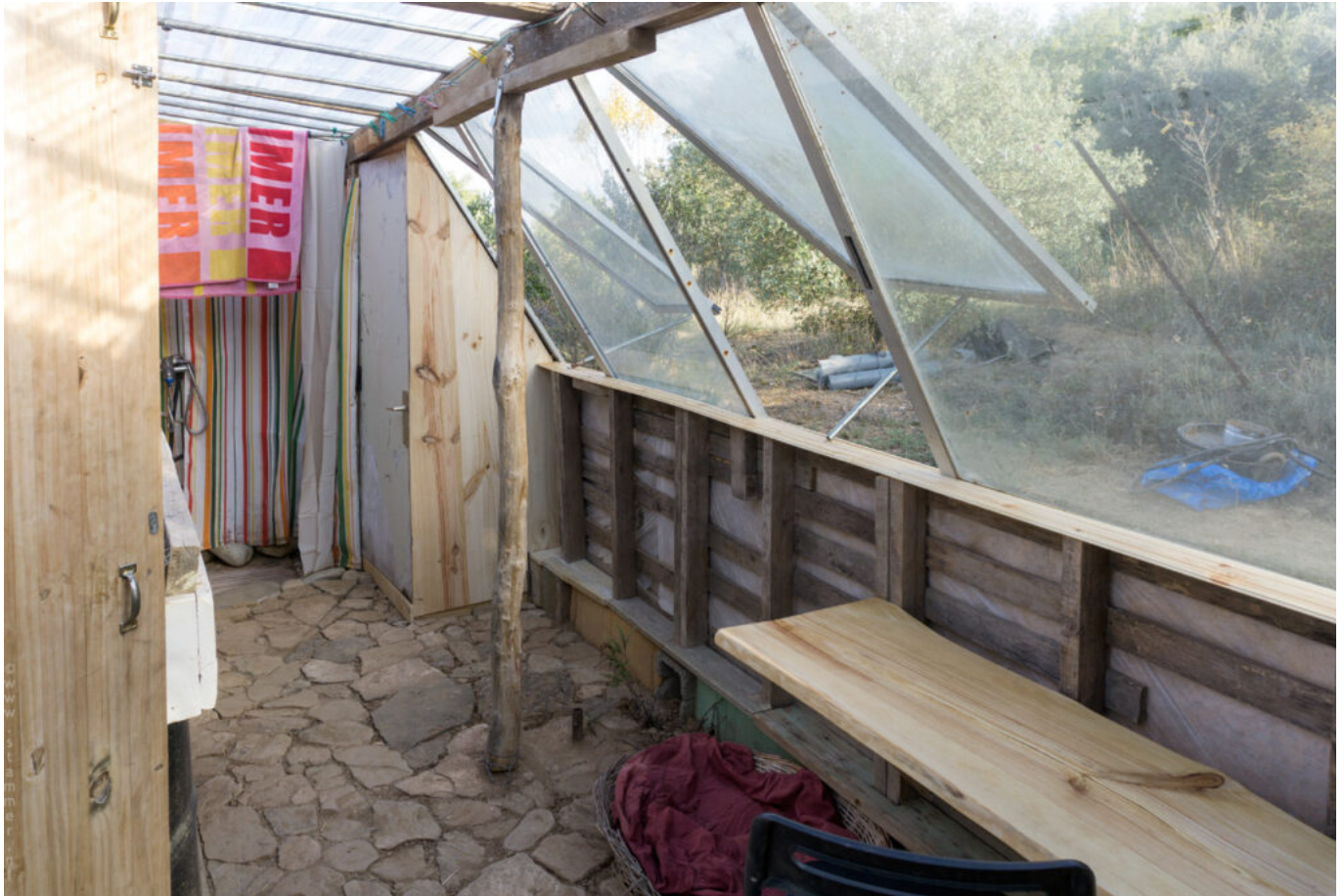
Interior of the new greenhouse, built with pallets, white cloth, wire mesh and adobe.
